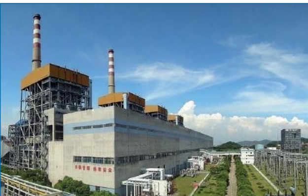
ZHUJIANG POWER COMPANY
